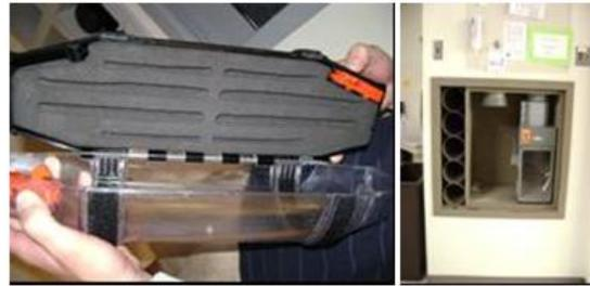
**Figure 8: The bullet carrier and bullet carrier system.**
