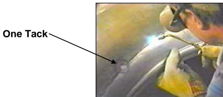
**Figure 2: A Welder Tacking Two Pieces of Metal Together** This process can be done many different ways depending on the preferred methods of the person doing it.
